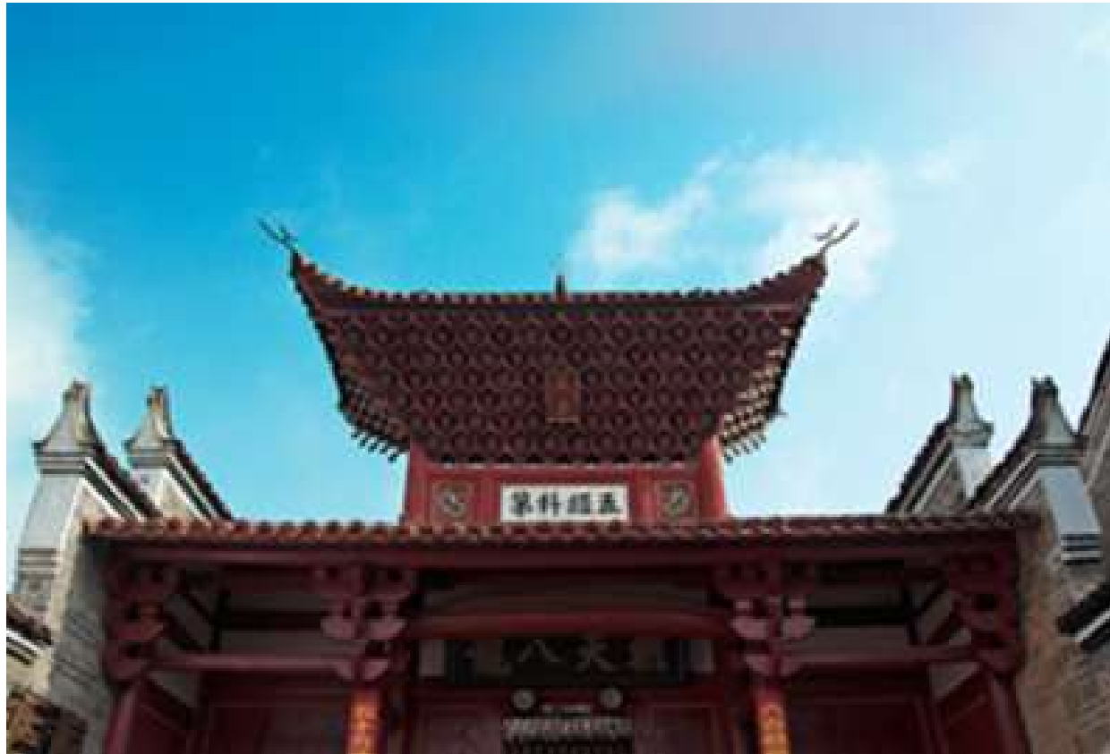
Ill. 3. Hanger with a groove and a tenon on the top floor of the Jiangxi Museum building. Source: author's photograph, 2020.
