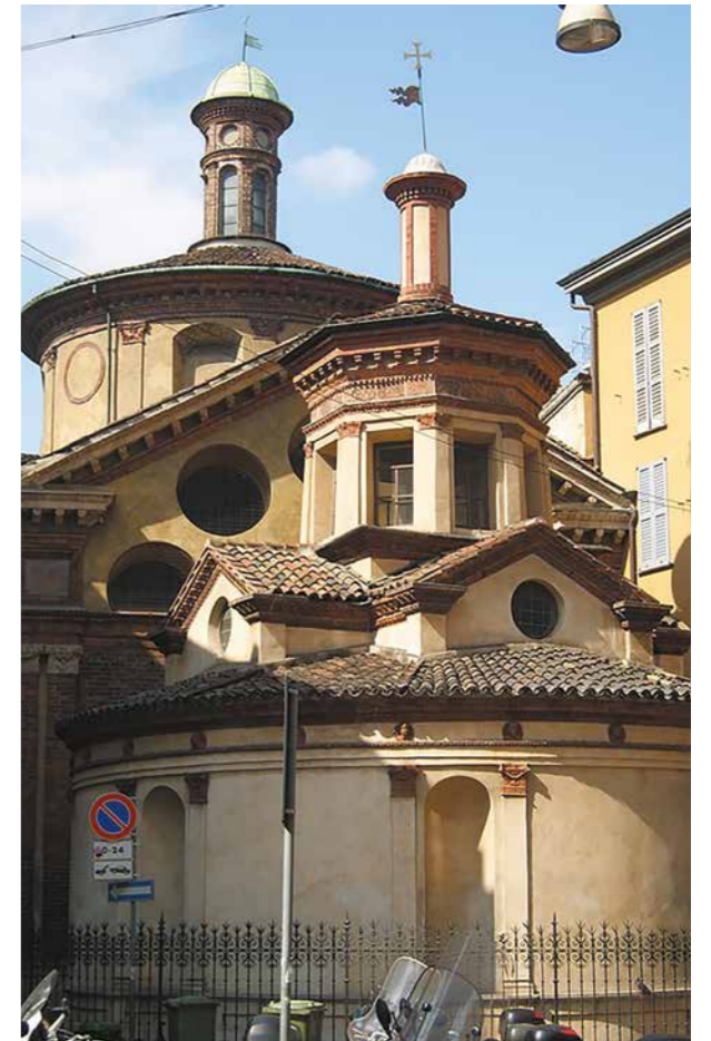
Ill.3. Chapel of San Satiro in Milan after its reconstruction by Bramante in the 1470s.
