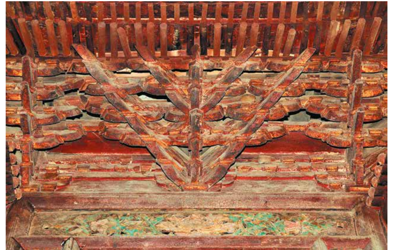
Ill. 8. Central dougong bracket at the Heavenly Palace Pavilion [7, p.39]
