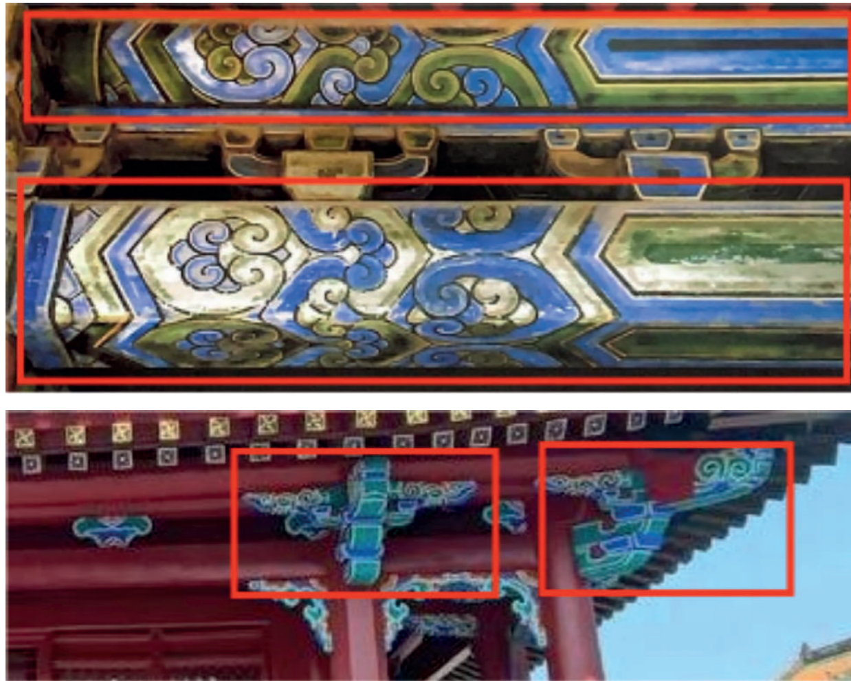
Ill. 7. At the top, there is a coloured painting on the outer cornice of one of the Shiwang Pavilions of the Forbidden City in Shenyang; it is made in the style of the Yau Mo type of the Xuanzi painted decoration. At the bottom, there is the Yau Mo type of the Xuanzi painted decoration on the Shenwu Gate of the Forbidden City in Beijing.
