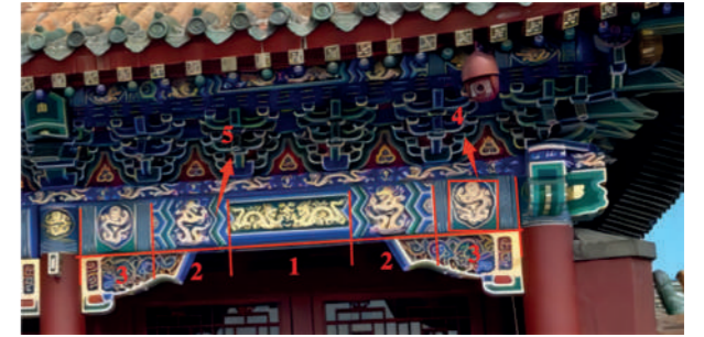
Ill. 8. The Dragon pattern of the middle Qing Dynasty (1736-1850) in the Jiguang Hall of the Forbidden City in Shenyang (1 — the central part of the beam painting; 2 — the intermediate part; 3 — the end part; 4 — "boxes"; 5 — fork lines).
