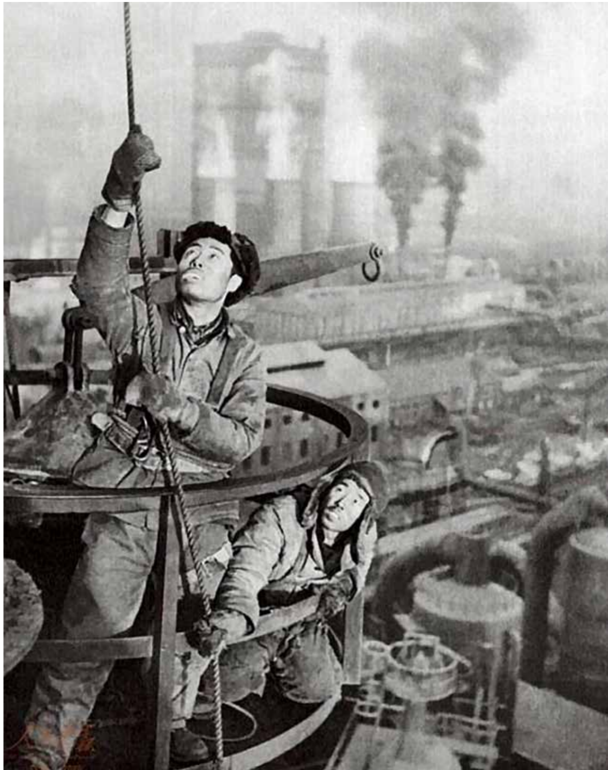
Fig. 4. Cai Shangxiang, Construction of the Anshan Steel Works , China magazine , 1951.
