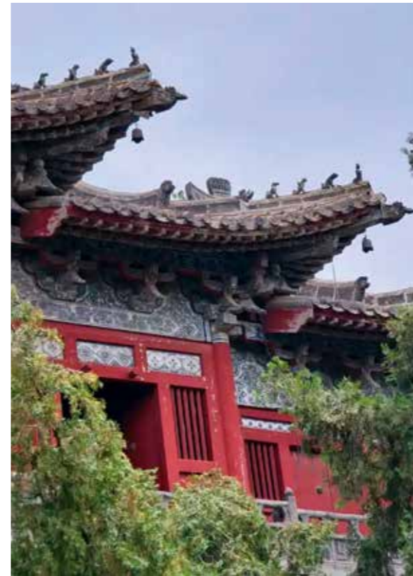
Fig. 3. Architectural polychrome painting ( jian zhu cai hua , 建筑彩画) on the structures of the Song mausoleum park in Gongyi (巩义宋陵公园). (图3: 图片是巩义宋陵公园中建筑上的建筑彩画。)
