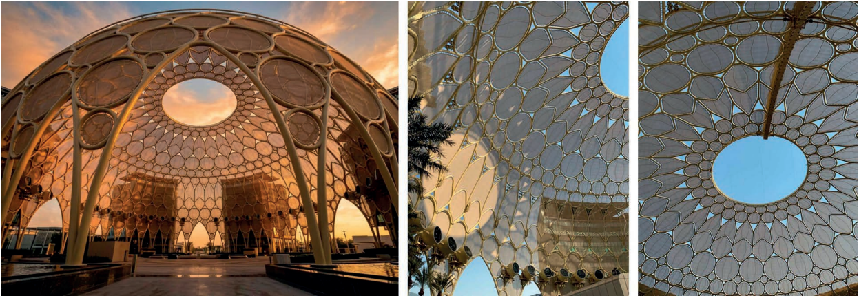
The dome of Al Wasl Plaza. Courtesy of START DXB (LEFT) and Open Space (MIDDLE and RIGHT)
